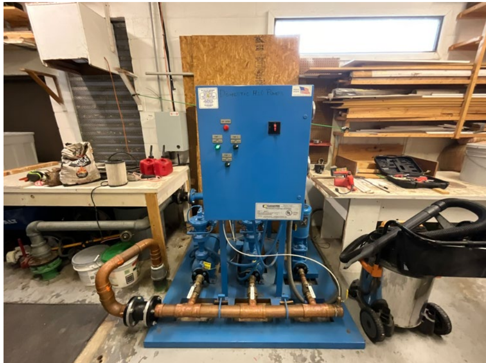
18. View of the domestic water pump system.
