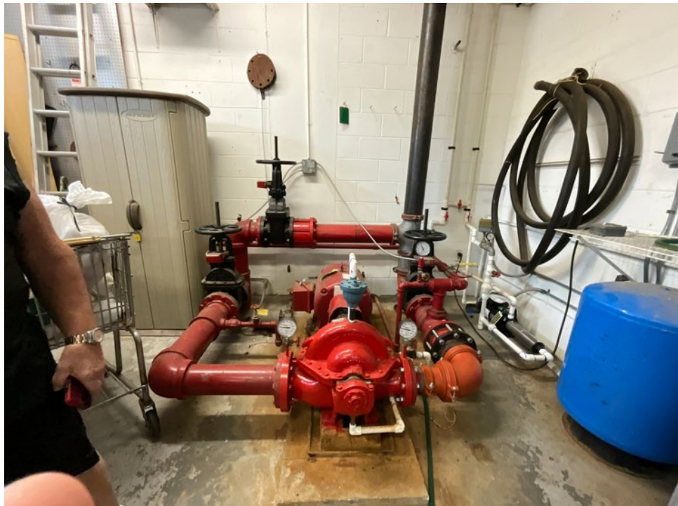
16. View of the fire suppression system pump.
