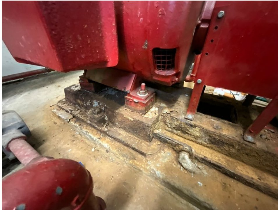
17. View of corrosion at the fire suppression system pump mounts.
