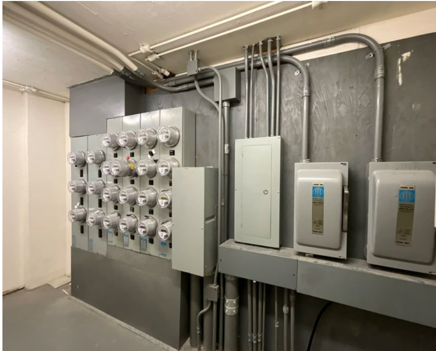
14. View of the typical meter stack, breaker panel, and sub-switches in the electrical rooms on floors 3, 6, and 9.
