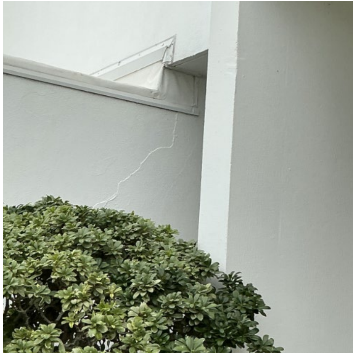
12. View of a stair-step crack in the ground-level CMU wall at the rear entrance.
