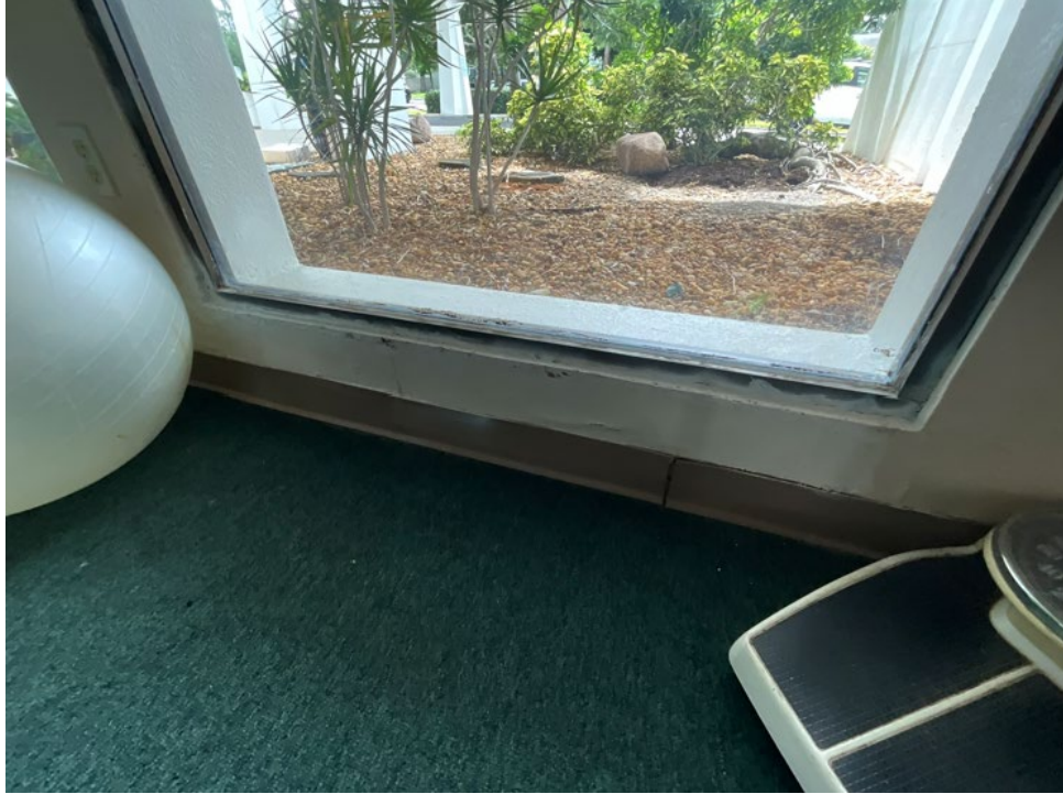
7. View of typical moisture intrusion at the common area windows.
