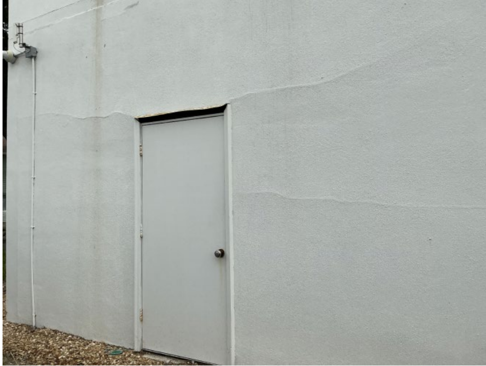
13. View of stucco cracks in the rear ancillary room wall.
